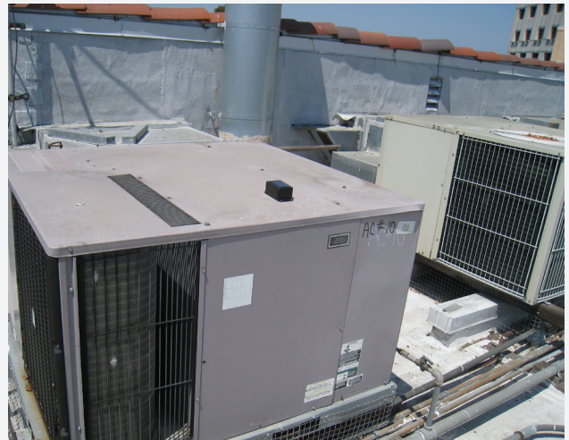
Figure 1 A solar-powered pervasive computer analyzing the condition of H/VAC equipment at Sentilla’s headquarters in Redwood City, California.
